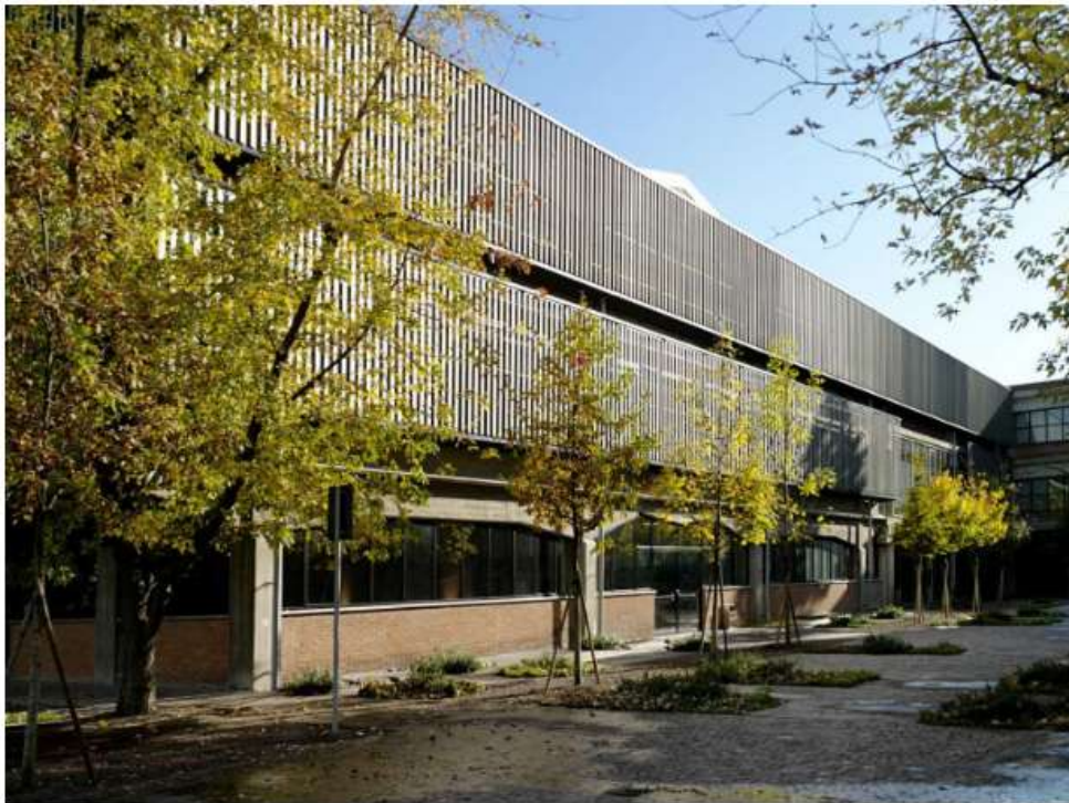
The Collezione Maramotti, as pictured in the March 2009 issue of Wallpaper* . The building was one of the first to contrast raw reinforced concrete with exposed brickwork on its exterior. Photography: Milo Keller & Julien Gallico
